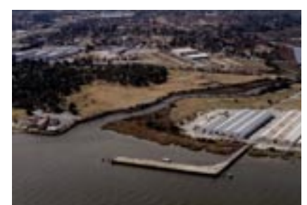
Pier Alpha at the junction of Noiset Creek and the Cooper River
