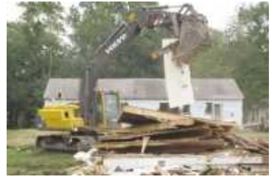
Deconstruction continues at up to 10 buildings a week.
